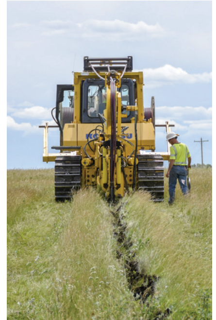
3C Foreman Doug Roethlisberger walks behind the plow train to make sure the cable is placed as planned. The plow train rumbles along at a steady pace, unless it hits rock and needs to slow down to slice through the barrier.
