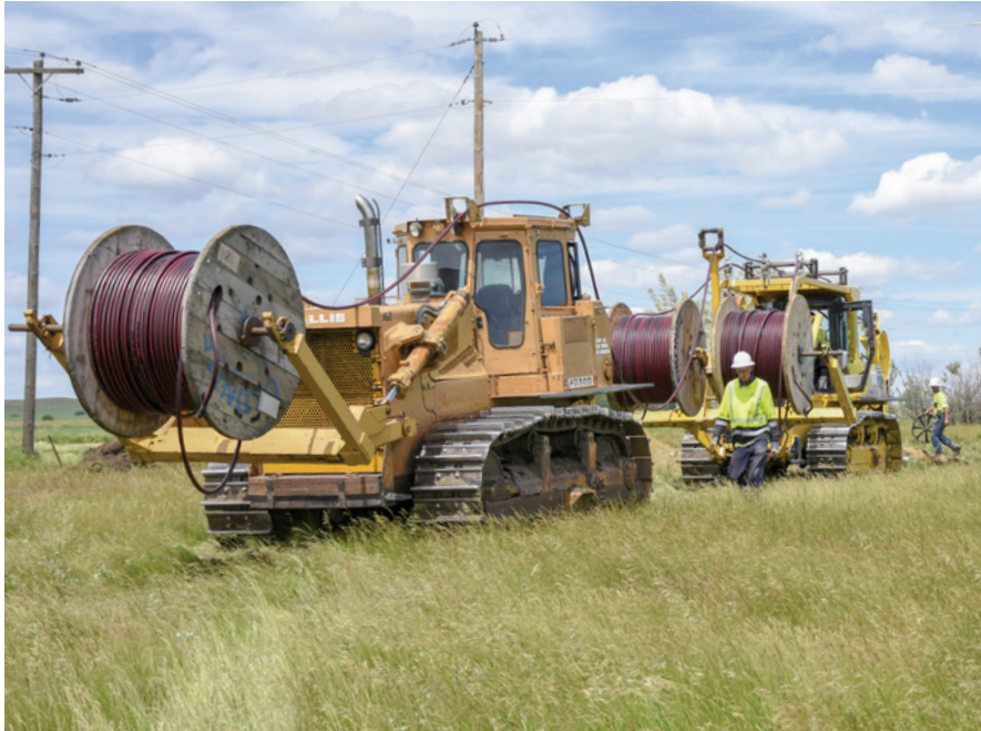
One of 3C Construction's specialties is its ability to plow cable relatively quickly with its plow train. Ron Roethlisberger, chief operations officer, hauls the equipment from site to site driving a semi that pulls a triple-axle tractor-trailer. Until you see the plow train in person, you may not realize the enormous size of the equipment — or the extraordinary narrow trench it leaves to lay cable. It performs a labor-intensive job, yet leaves a minimal footprint. Plowing cable for long stretches is an efficient and economical process.
