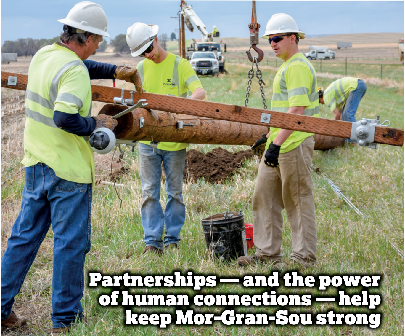
Allen Scherr, Corey Eberle and Ethan Volk (a former employee with 3C) work on dressing a new pole, as Mor-Gran-Sou line crews set replacement poles in the background.
