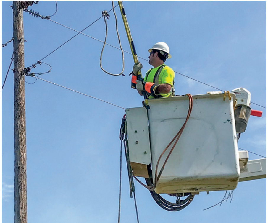
Mor-Gran-Sou Journeyman Lineman Cody Graetz grounds the line on both sides to change out a pole.
