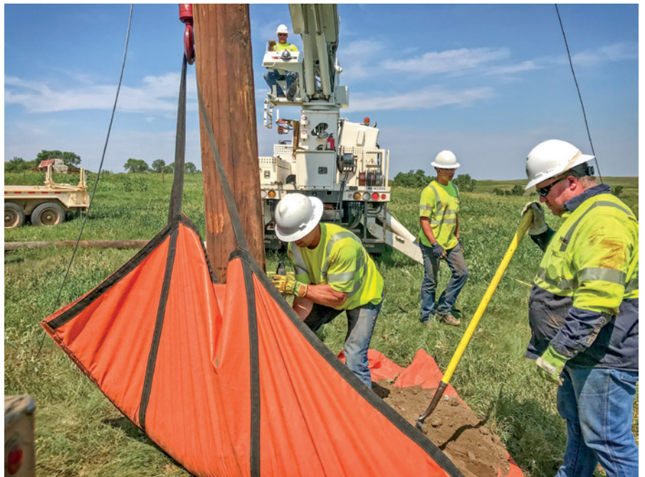
NDAREC Safety Instructor Steve Homes (right) watches Mor-Gran-Sou Apprentice Lineman Kale Ohlhauser tamp a pole.
