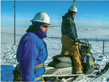
Lead Men Clint Begger (snowmobile) and Gary Fitterer restoring electric service after the January 2010 storm.
