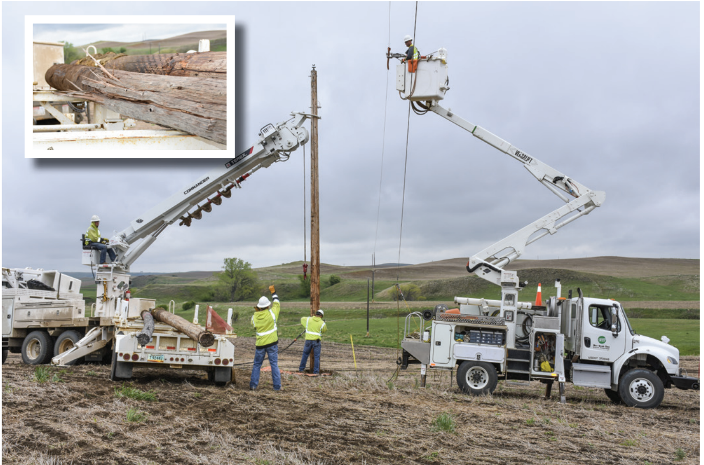
From left: Journeyman Lineman Blake Reis (operating digger-derrick), Leadman Clint Begger (holding plumb bob), Journeyman Lineman Brady Zachmann (tamping dirt) and Leadman Jason Jahner (waiting to reattach power line, from bucket) worked the line hot to avoid disrupting power to the member.
