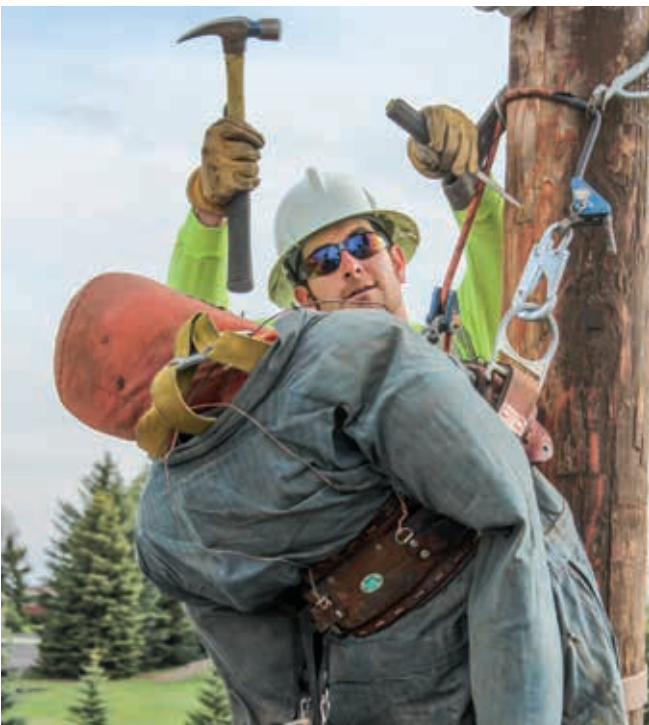
Journeyman Lineman Cody Graetz pounded a screwdriver into the pole to secure his rope, before threading it around the stranded mannequin.
