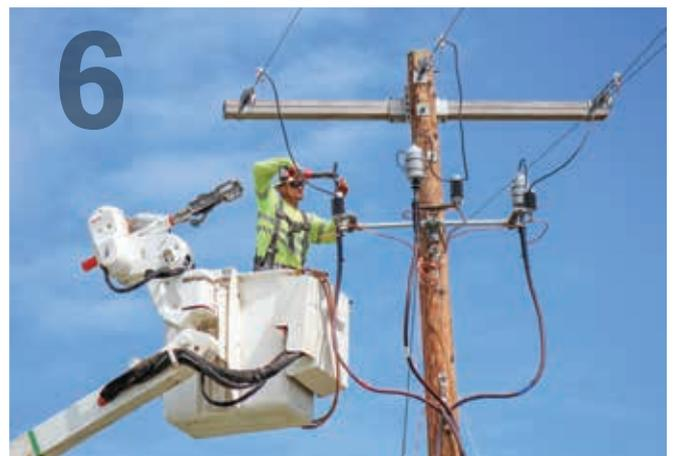
6. Journeyman Lineman **Brady Zachmann** crimped the terminator and added cover-up. When the new overhead to underground transition is complete, all energized parts will have insulated cover-up to protect birds and other wildlife from being electrocuted and possibly causing a power outage.
