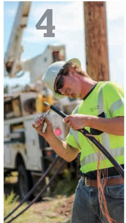
4. Where the underground powerline meets the overhead distribution to the south, another line crew prepares the cable. Journeyman Lineman **Blake Reis** removed the jacket, cleaned the cable and added a terminator.
