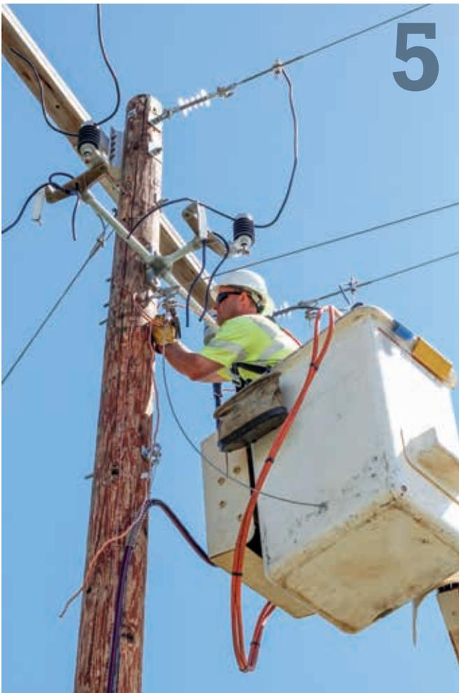
5. Once the underground cable was fed up the pole and connected to the de-energized overhead system, Leadman **Jason Jahner** used a hydraulic compression tool to attach the equipment grounds. Then he applied U-Guard™ to protect the cable from the elements.
