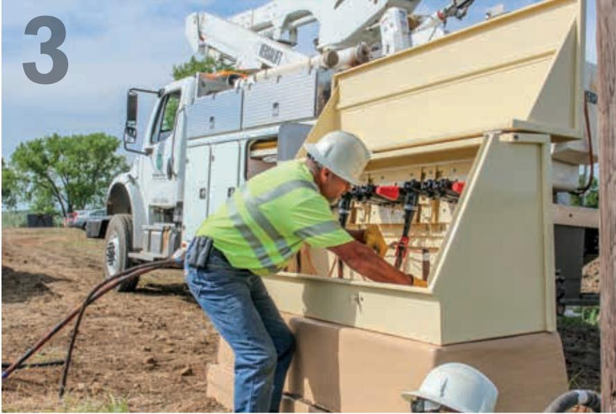
3. Once prepared, the cable will be enclosed in a locked vault. Trenched four feet below the earth's surface, the new cable runs south for a little more than half a mile. Cottonwood trees have been damaging the overhead power lines during windy conditions over the years. The new underground cable will improve reliability to the area. Here, General Foreman **Doug Nagel** connects cable in the vault.
