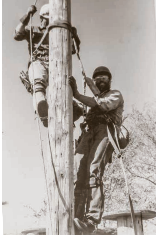
Prior to June 2014, OSHA didn’t require linemen to wear a safety belt while climbing; they only had to wear one while working in the air. Here, former Mor-Gran-Sou Electric Lineman Terry Kraft (bottom) prepared to free-climb a pole.
