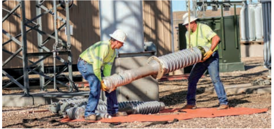
Fort Yates Area Foreman Brent Alkire and General Foreman Doug Nagel prepare the parts and pieces needed to be added to the new transformer once placed on the concrete pad. Once "dressed" with all accessories and oil, the new transformer will weigh 130,000 pounds.
