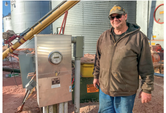
Mark Doll relies on electric service to power his grain-drying system and make this late-season harvest possible.
